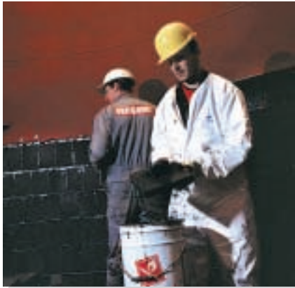
Chimney flue cans are pre-lined on ground level.
