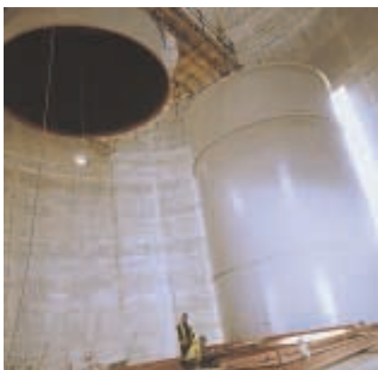
A pre-lined flue can enters the chimney.
