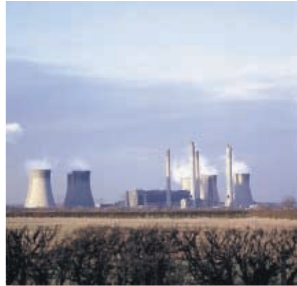
West Burton Power Station
