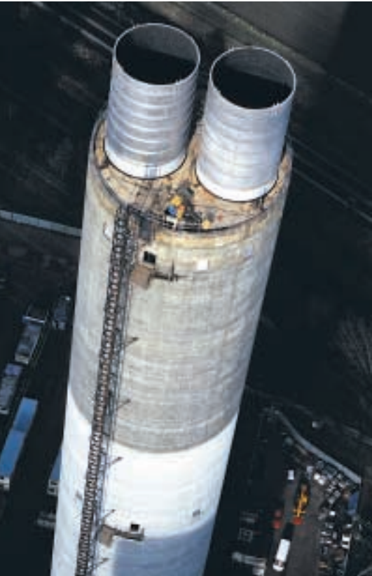
One of the new, 200 m high FGD chimneys.
