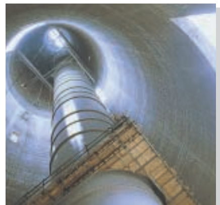
A chimney flue during the erection process.
