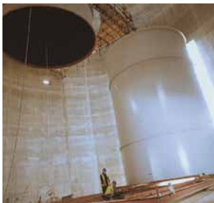
A pre-lined flue can enters the chimney.
