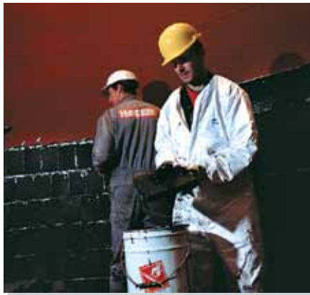
Chimney flue cans are pre-lined on ground level.
