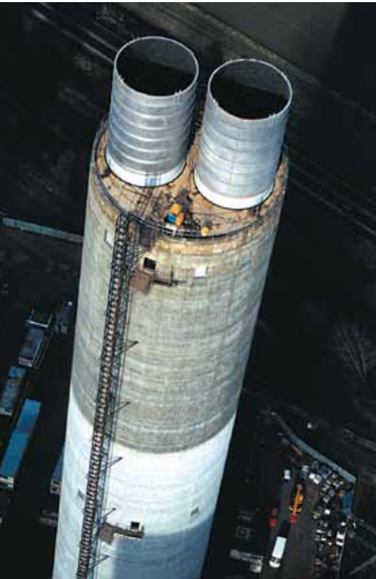
One of the new, 200 m (656 ft) high FGD chimneys.
