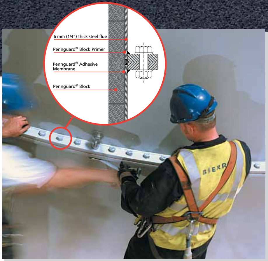
The chimney flue cans are installed using bolted flanges.
