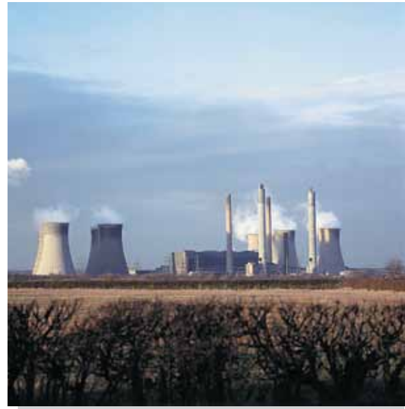
West Burton Power Station
