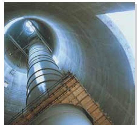
A chimney flue during the erection process.
