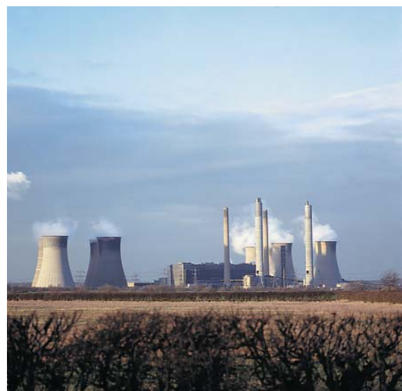
West Burton Power Station
