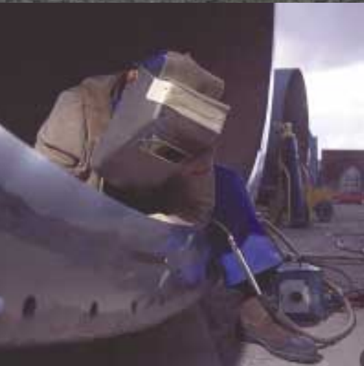
Welding of alloy protection strips.
