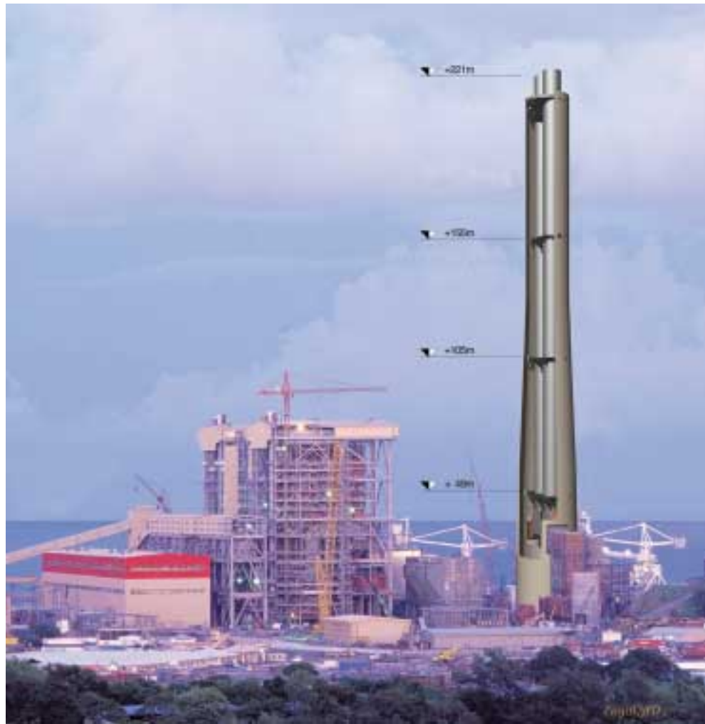
The reinforced concrete windshield contains two steel flues.
