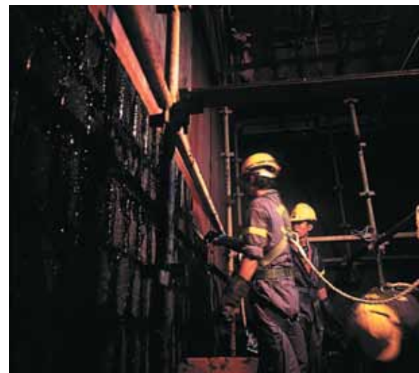
Application on the lower rectangular section of one flue.
