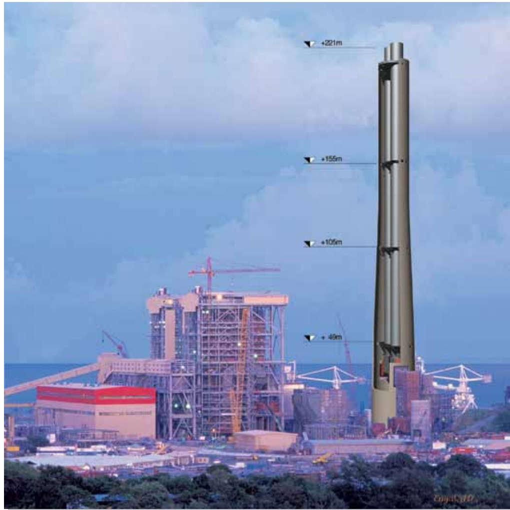
The reinforced concrete windshield contains two steel flues.
