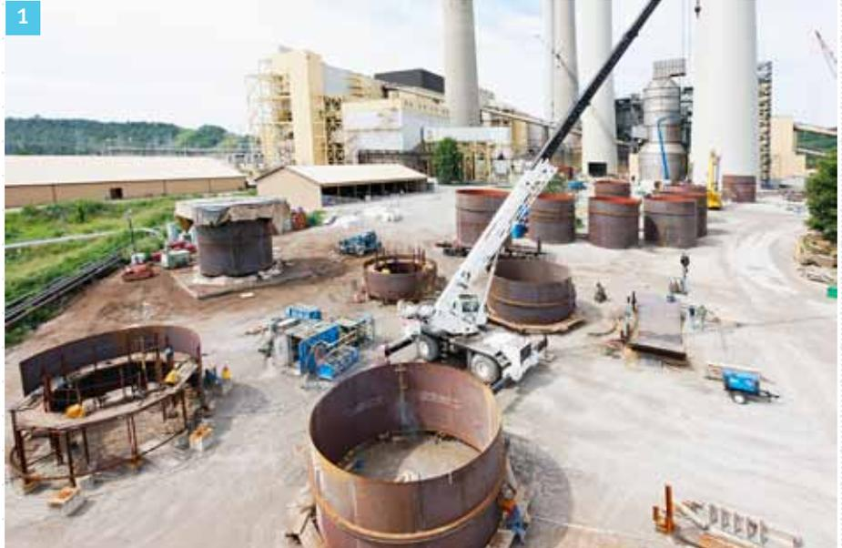
1. The steel flue diameter of the Unit 1 chimney is 6.40 metres. The Unit 2 steel flue is 8.24 metres in diameter. Karrena decided to pre-fabricate steel flue sections on site, close to the new chimneys. The grit blasting required for the Pennguard® Block Lining System, as well as the application of Pennguard® Block Primer, were also performed on ground level.
