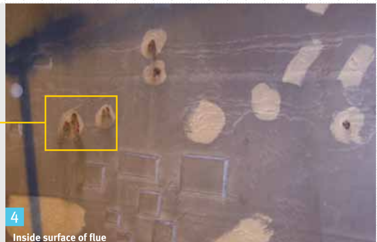
Corroded spots repaired with new coating, corroded again
