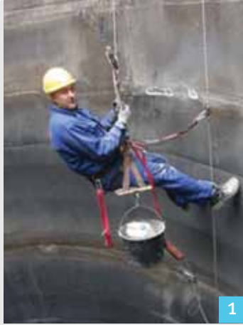
Repair of corroded steel areas
