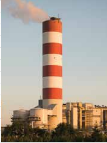
FGD wet stack with two steel flues
