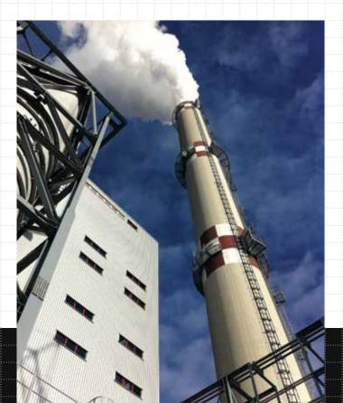
As a result of the warming effect of the Wet Booster Fans and the limited temperature loss by the flue gas flowing through the Pennguard lined chimneys, the condensate formation in the Rovinari wet stacks will be reduced to effectively zero under most operating conditions.
