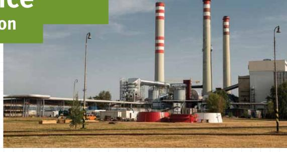
Lignite fired power station renews its flue gas desulphurization system and converts its existing chimney to a Pennguard<sup>TM</sup> lined wet stack
