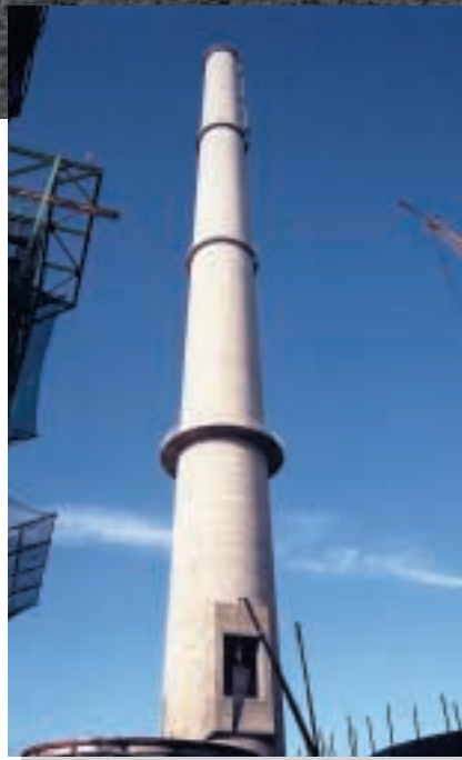
Unit 6 chimney under construction
