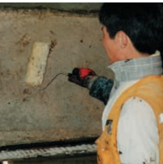
Penntrowel Epoxy Primer seals the concrete surface
