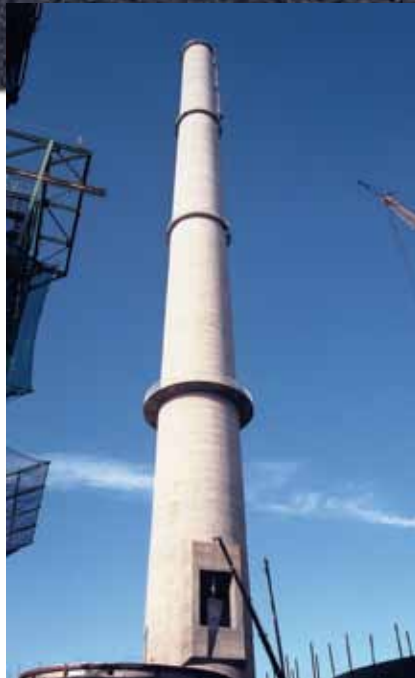
Unit 6 chimney under construction
