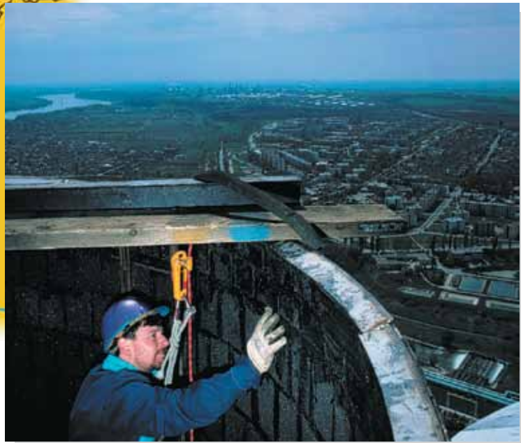
The top of each flue sticks out of the concrete shell and is especially vulnerable to cold spots.
