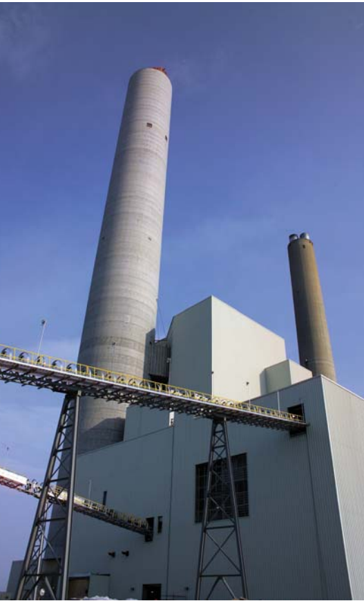
The building housing the FGD and wet ESP, with the new chimney.
