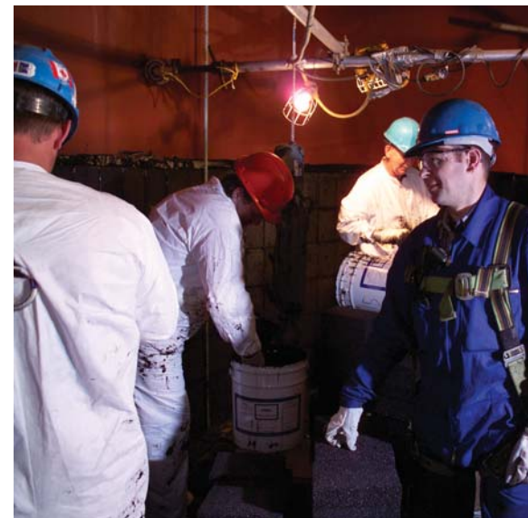
The lining installation process was completely supervised by Hadek Quality Inspectors.
