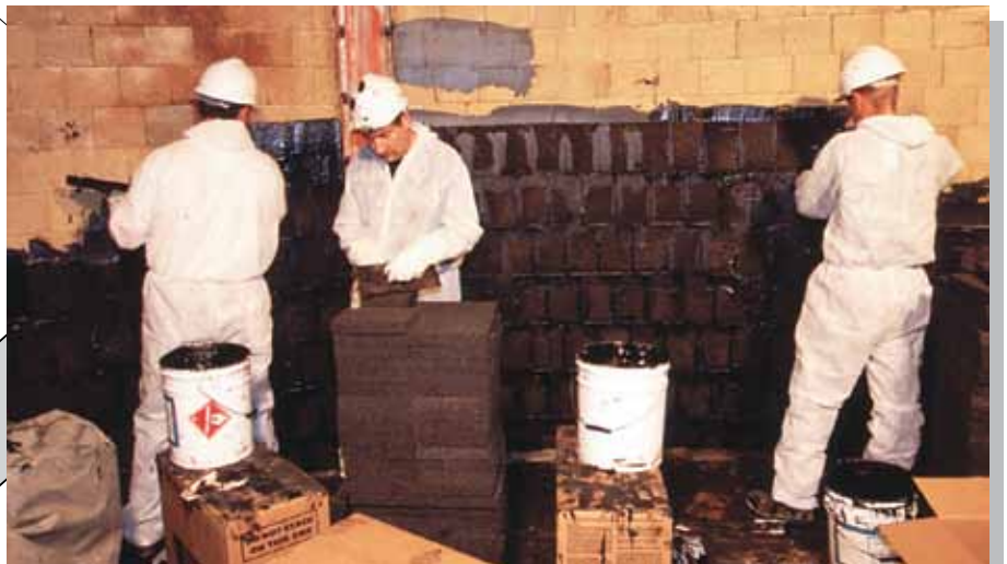
Experienced brick layers apply the Pennguard® lining.
