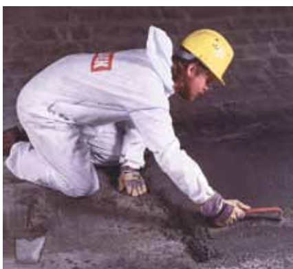
The chimney floor receives an additional layer of acid resistant cement.
