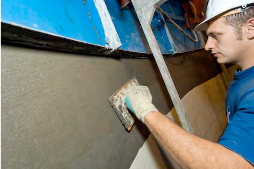
Picture 2 Screeding the surface
