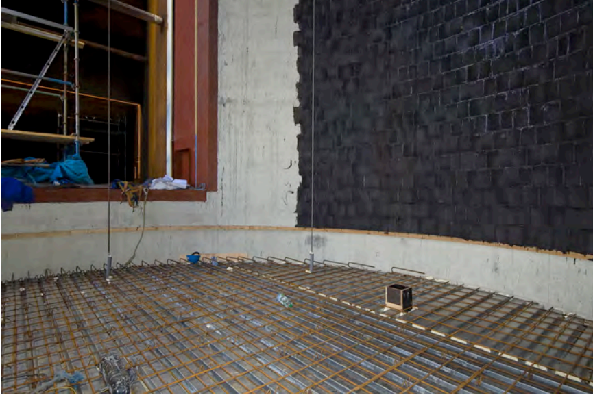
Picture 6 Floor, just below breaching
