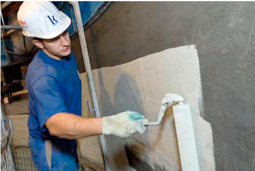
Picture 3 Applying vapor retaining primer
