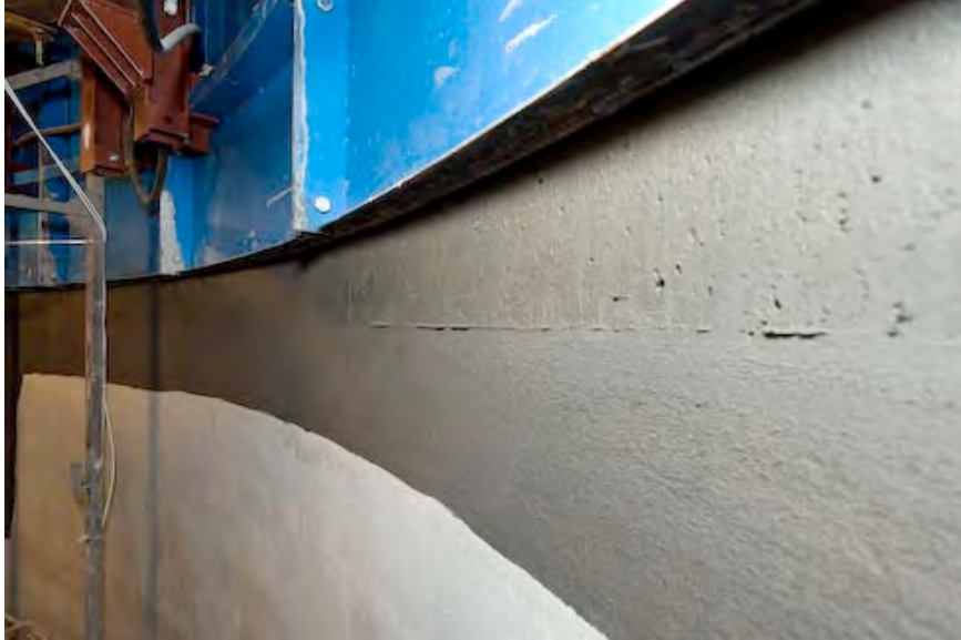
Picture 4 Concrete out of slipform, screeded concrete, primed concrete.
