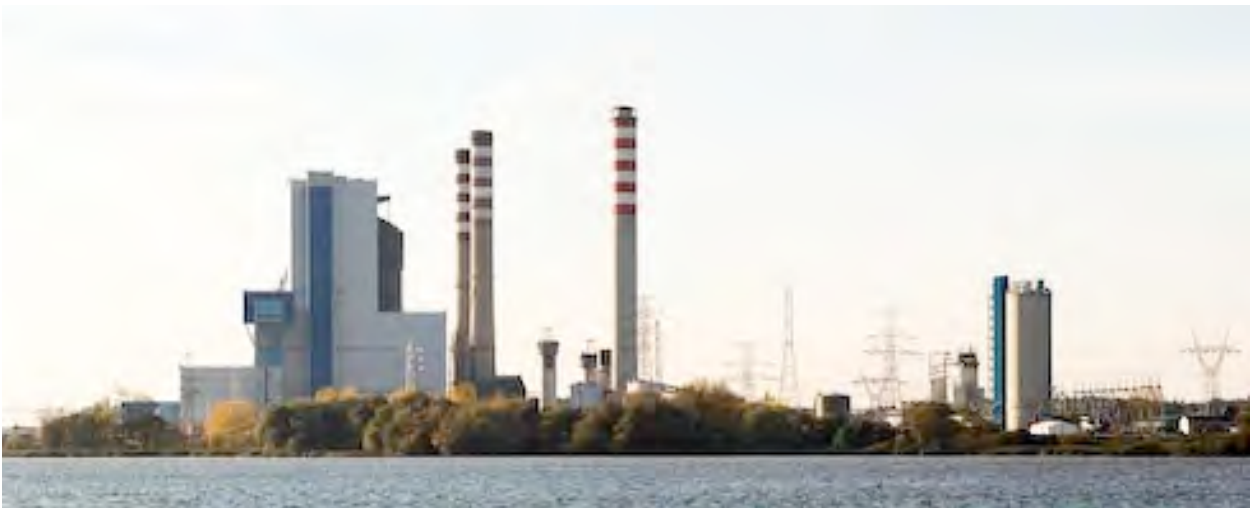
Picture 7 Power station with two new chimneys going up between existing
