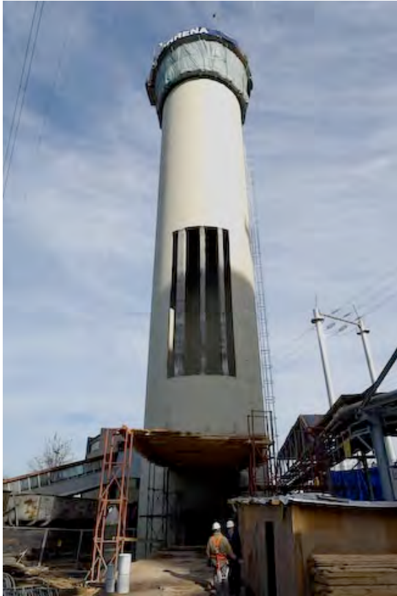
Picture 1 Slipforming of the concrete shell
