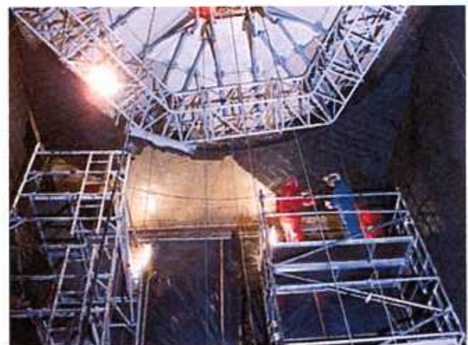
Figure 15 – Lining application at inlet section
