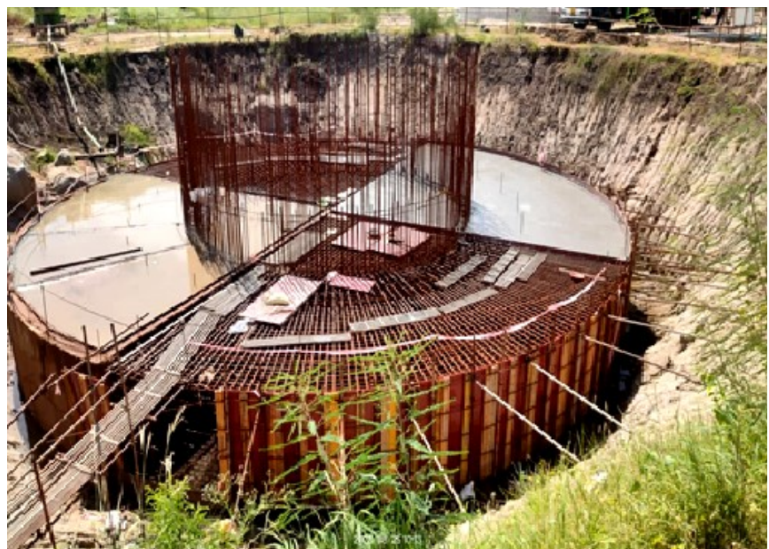
Figure 1: Chimney raft concreting
