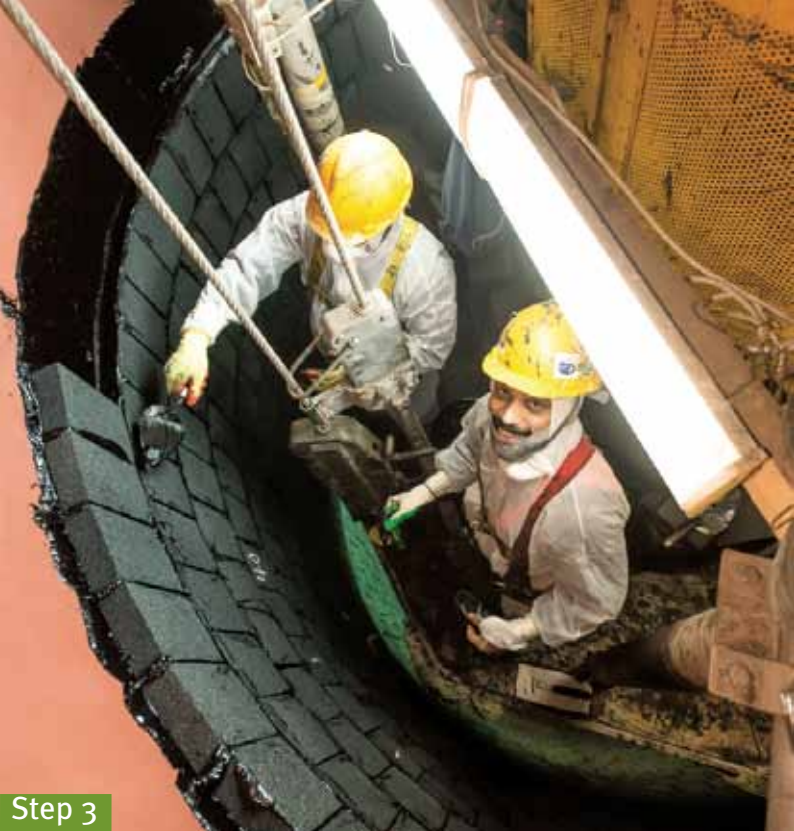
Installing the Pennguard® lining
