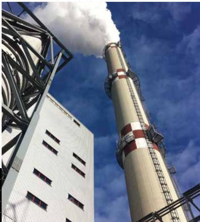
As a result of the warming effect of the Wet Booster Fans and the limited temperature loss by the flue gas flowing through the Pennguard lined chimneys, the condensate formation in the Rovinari wet stacks will be reduced to effectively zero under most operating conditions.
