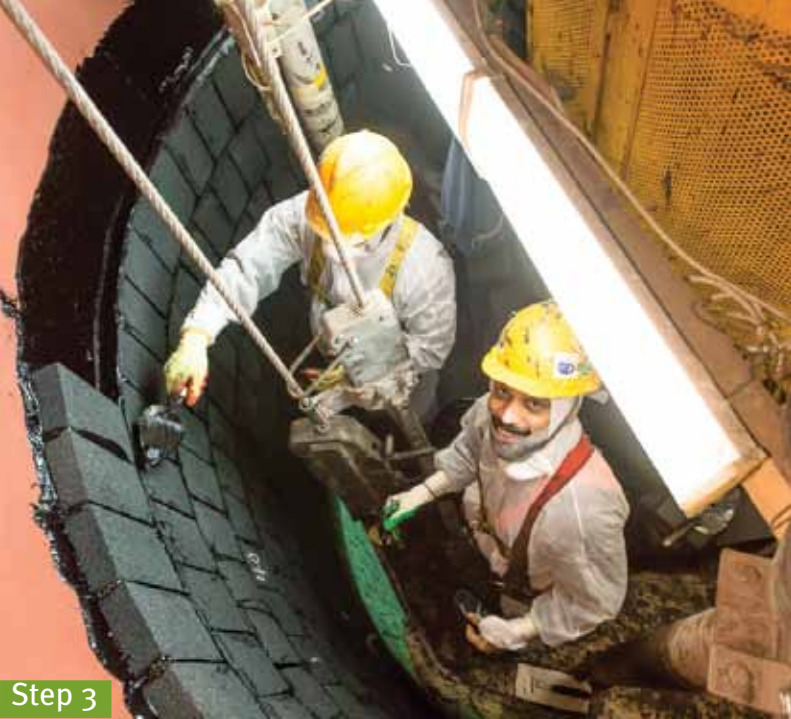
Installing the Pennguard® lining
