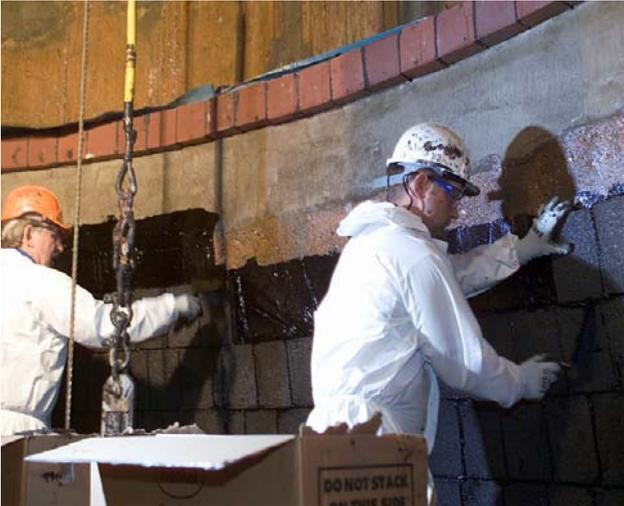
Figure 12: Installation of the Pennguard® lining
