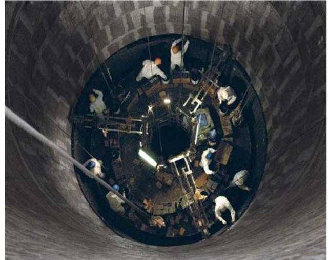
Figure 15: Installation of the Pennguard® lining in one flue took 30 days
