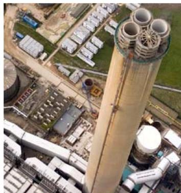
The existing 200 m high chimney was built in 1965 with 4 concrete flues, each with a diameter of 8 to 7 m and each internally lined with ceramic brick. The ceramic brick is divided in sections of about 10 m high and built up from the corbel supports in the concrete flues (Figure 2).
