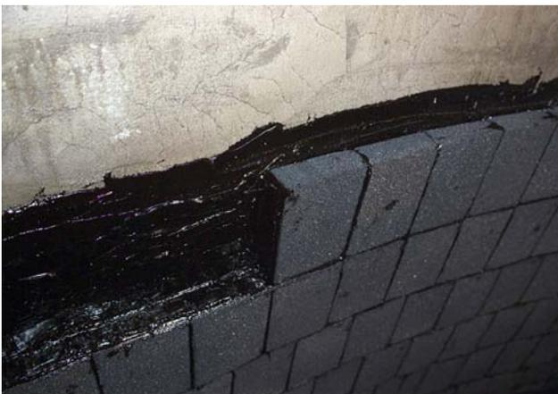
**Figure 4 A: Pennguard® lining on concrete,**
